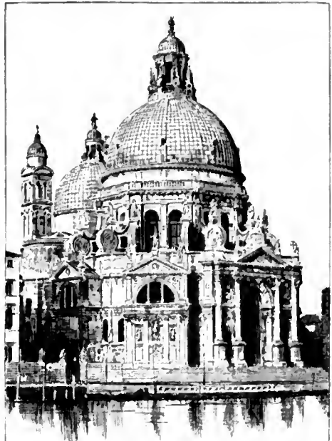
Italian Architecture.—Church of Sta. Maria della Salute, Venice; constructed 1632.
